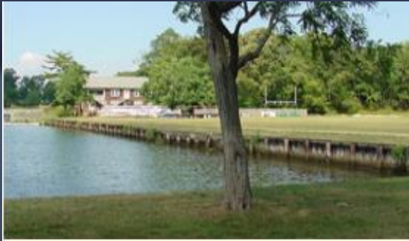
The St. John's College living shorelines site before the living shorelines were installed.
